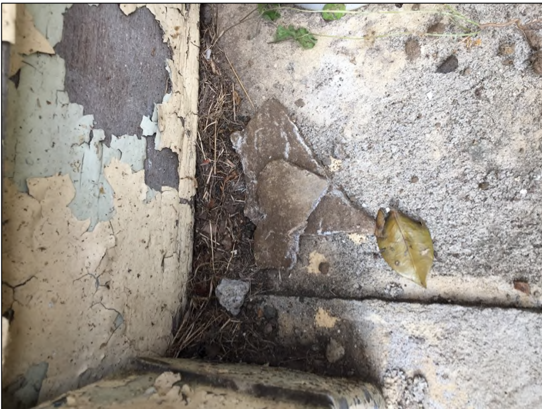
Photograph 8: Pieces of asbestos containing material identified at sample location 10.
